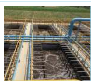
SET-Diffused Aeration with Lifting Arrangement for ETP
