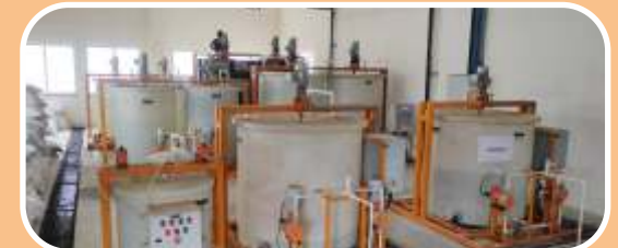
Automated Chemical Dosing System
